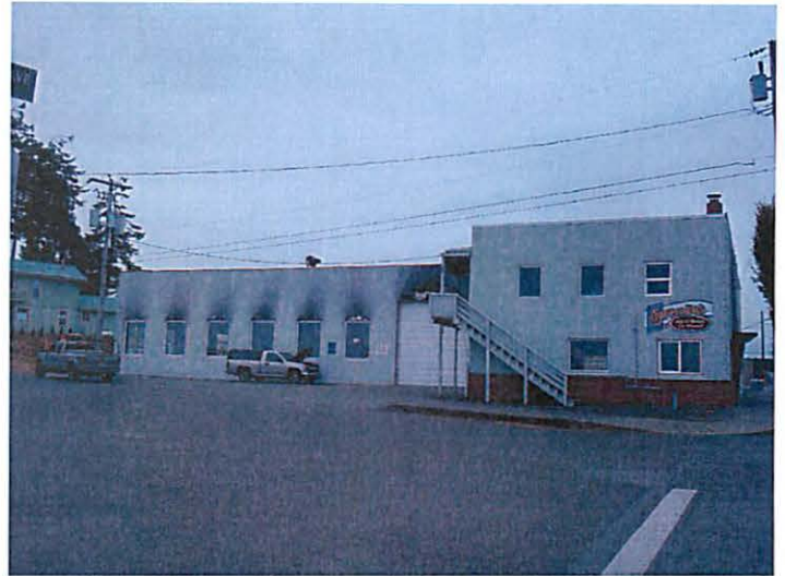
View of West Elevation facing North Main Street
