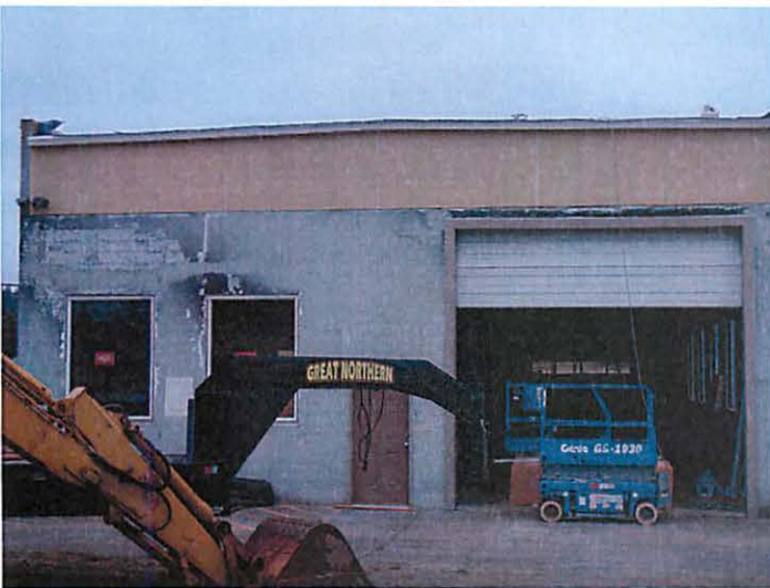
View of North Elevation
