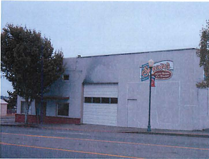
View of South Elevation facing Newmark Avenue
