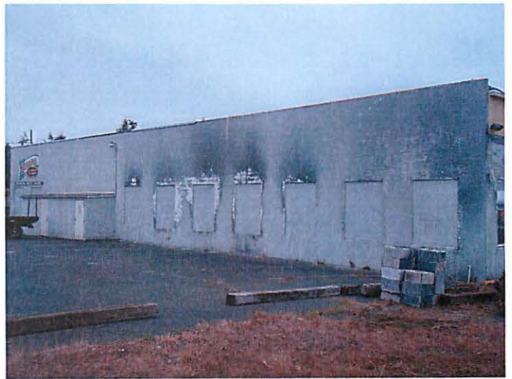
View of East Elevation facing off-street parking lot
