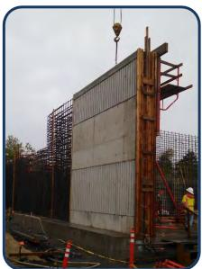
Pictured to the left is the first wall on the S Empire Blvd side of the project. Pictured above depicts the amount of rebar used to insure long term structural stability.
