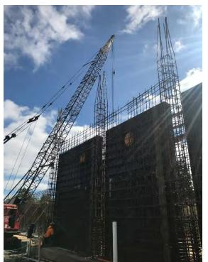
Nice weather has brought nice progress on the Wastewater Treatment Plant 2 project. Walls are going up! Crews have been working hard to get all the rebar placed and ready for nice days to have concrete pours.
