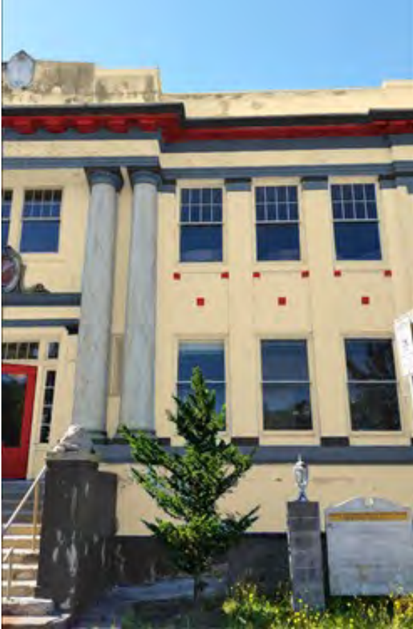
Central Ave View
