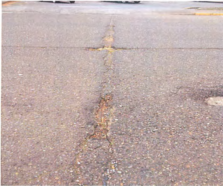
Longitudinal cracking of concrete surface below the asphalt paving.
