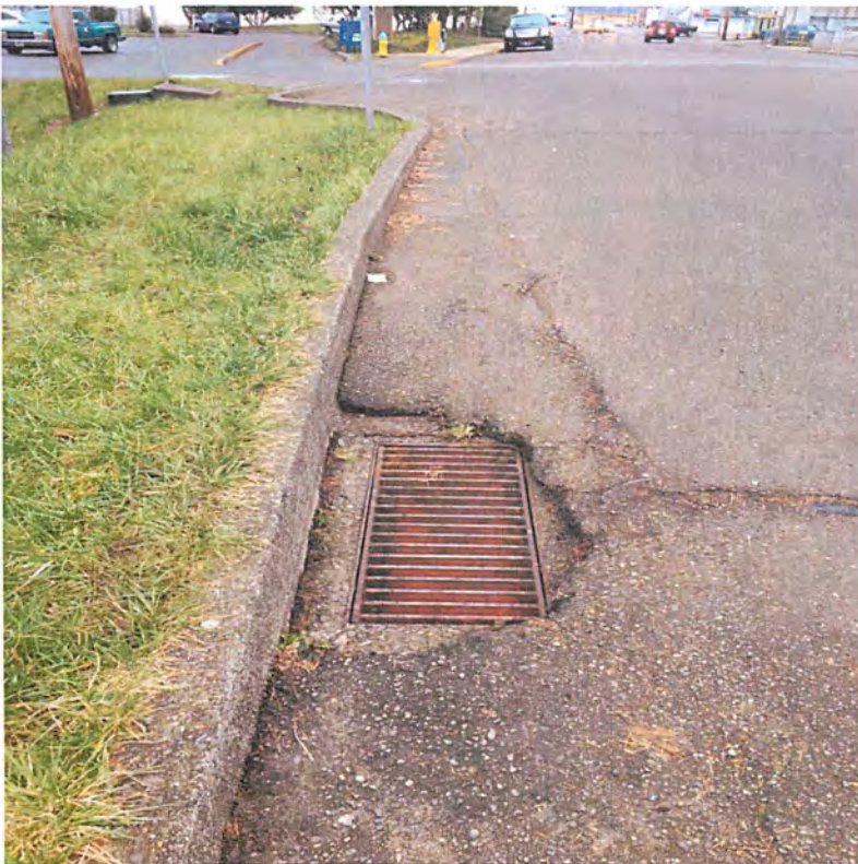
Catch basin condition from previous overlay of Golden Ave.
