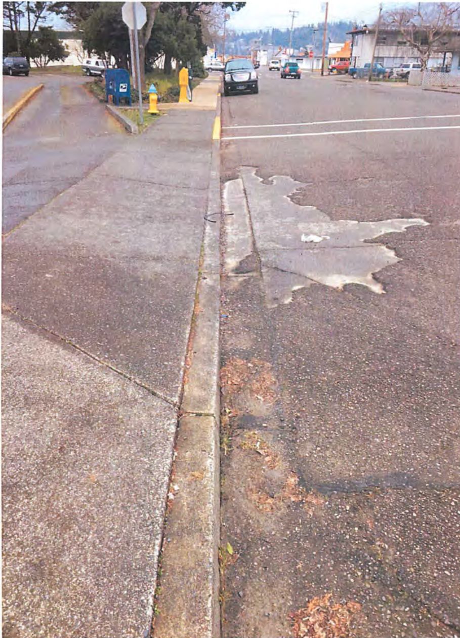
More delamination of asphalt from the concrete surface underneath.
