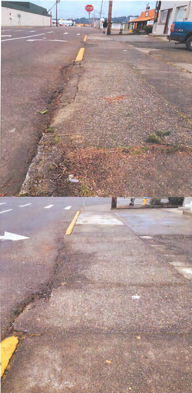
The pictures above shown distress and ponding in driveways on south side.
