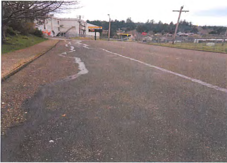
The picture above shows the trench repair the goes the entire length of Golden Ave. from 4 th street to 7 th Street.
