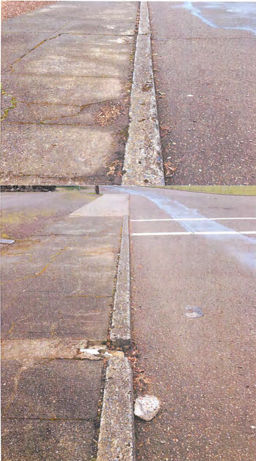
The pictures above show the condition of the curb & gutter.
