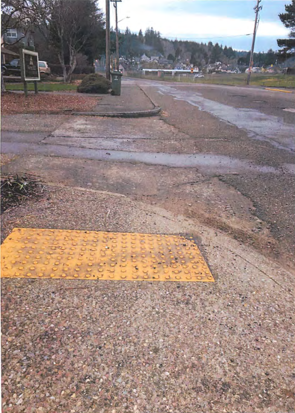
This is actually an alley that would require ADA ramps or converted to a driveway approach.
