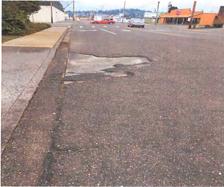
Golden Ave. pavement delamination.
