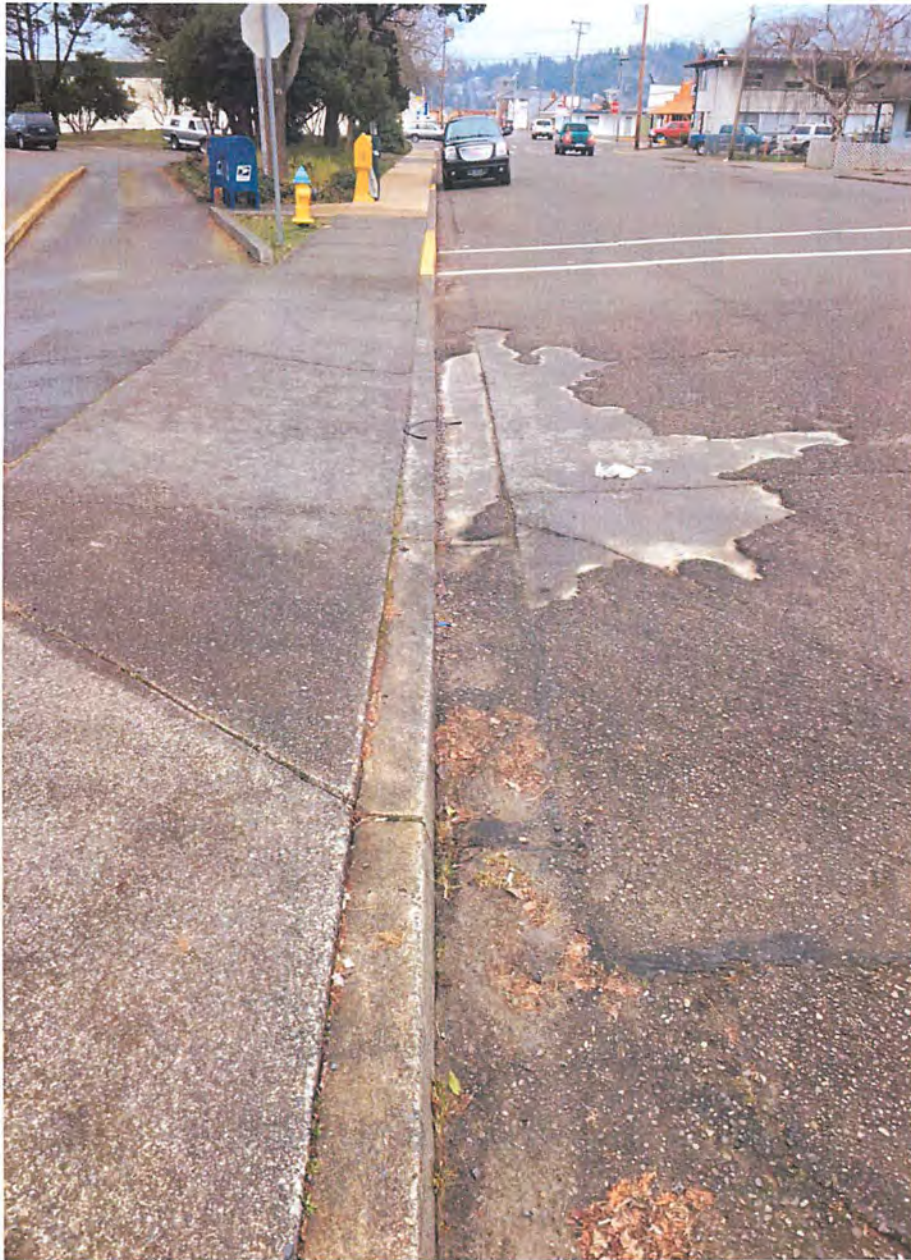
More delamination of asphalt from the concrete surface underneath.
