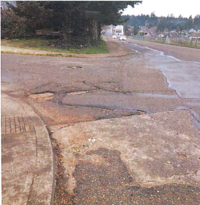
The picture above shows the condition of the intersection of Golden Ave. & 5 th Street.
