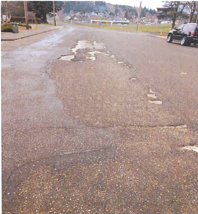
Golden Ave. looking west from 4 th Street, pavement delamination at centerline.
