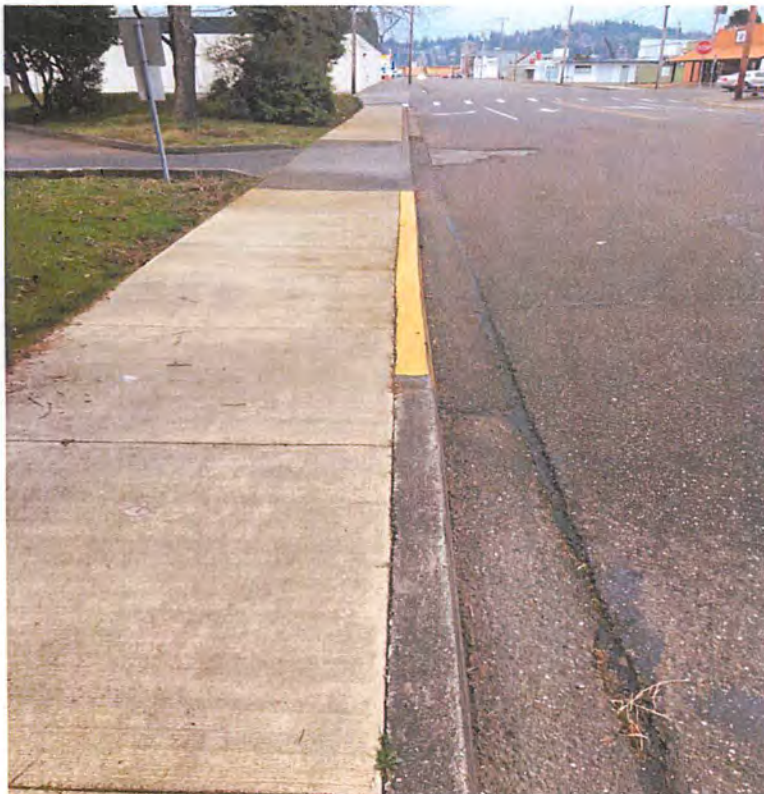
Golden Ave. looking east in front of Post Office.
