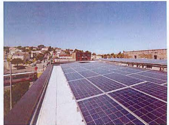
A vegetated roof on the Bayview library filters stormwater on-site and PV panels provide renewable energy. Hacker Architects.
