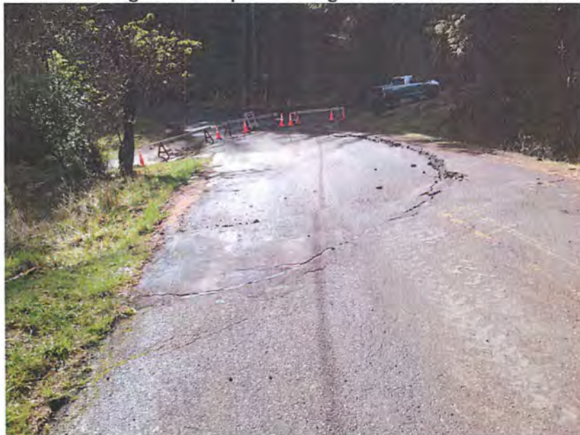
Photo illustrating headscarp extending across the entire road width.
