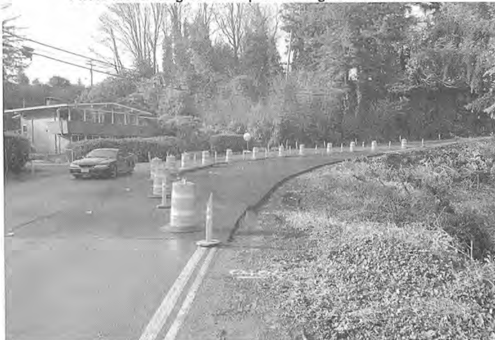
Photo illustrating headscarp extending into travel lane.
