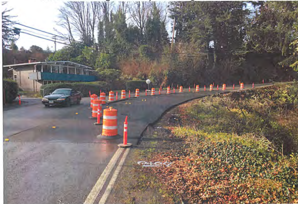
Photo illustrating headscarp extending into travel lane.
