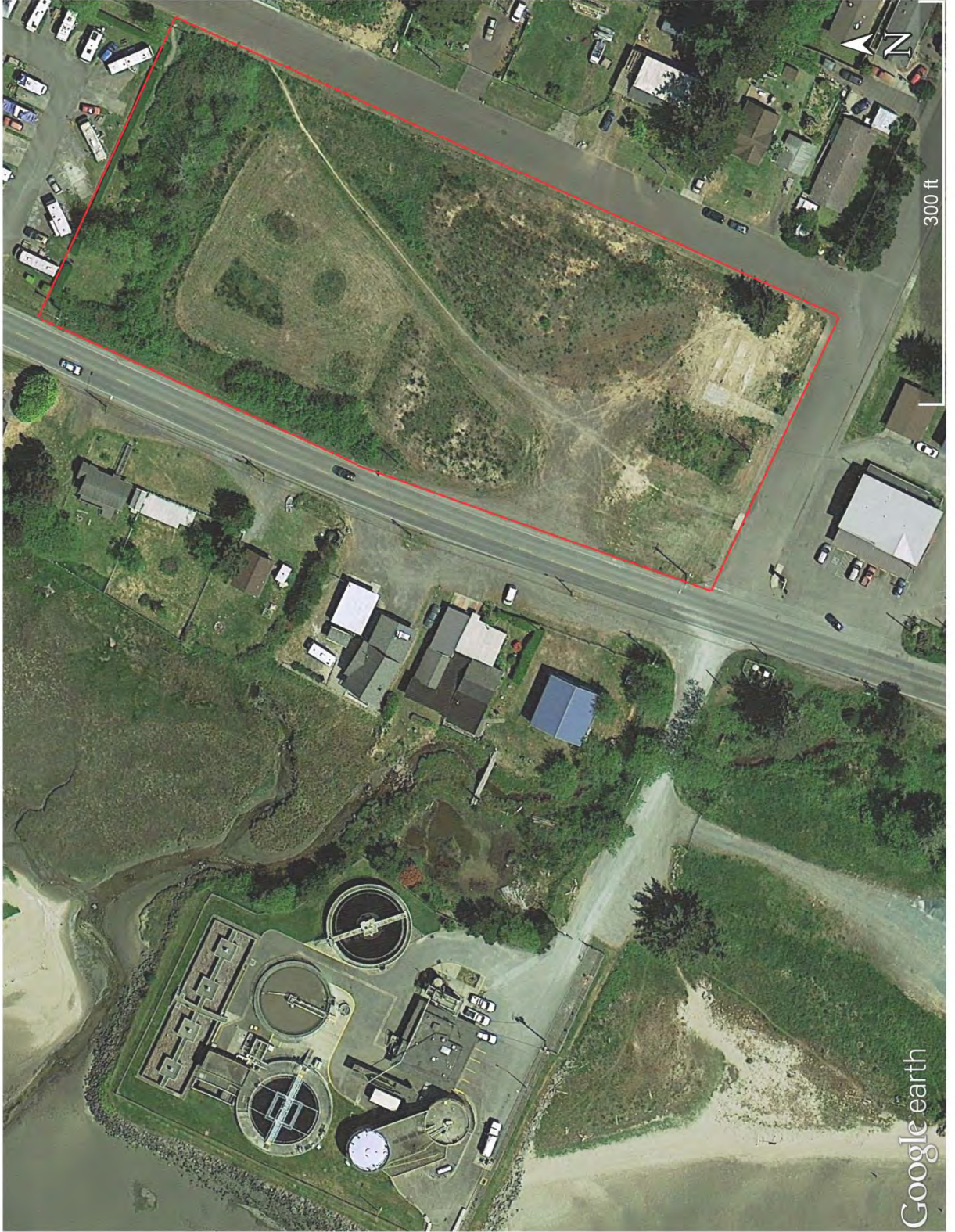
AERIAL OF NEW CB2 SITE
