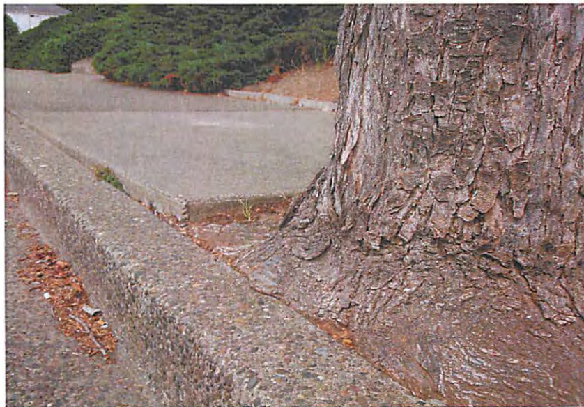
Tree root damage caused to sidewalk
