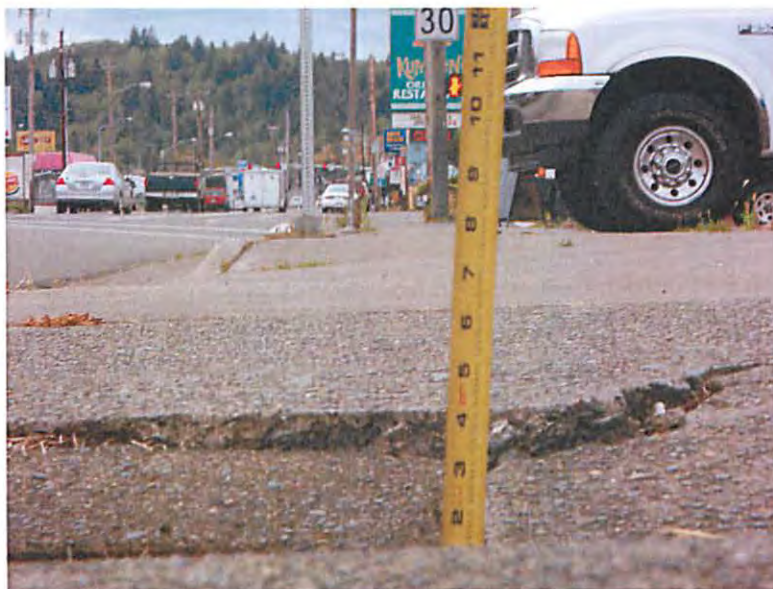
Vertical separation along cracks
