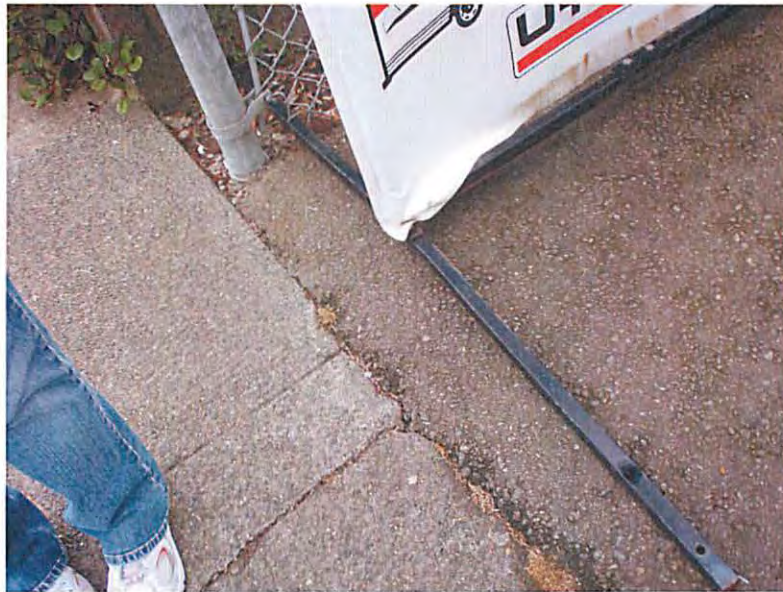
Vertical separation at the score line.
