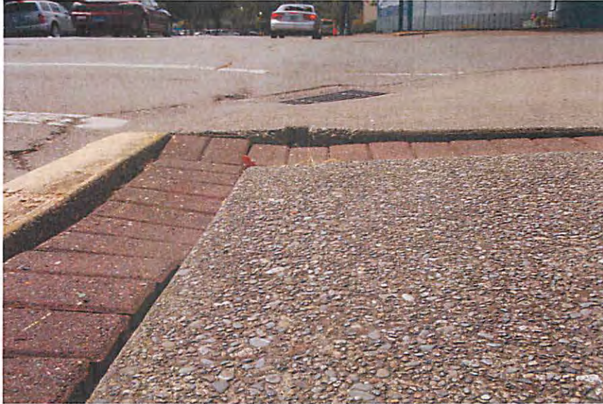
Brick separation along tree wells.
