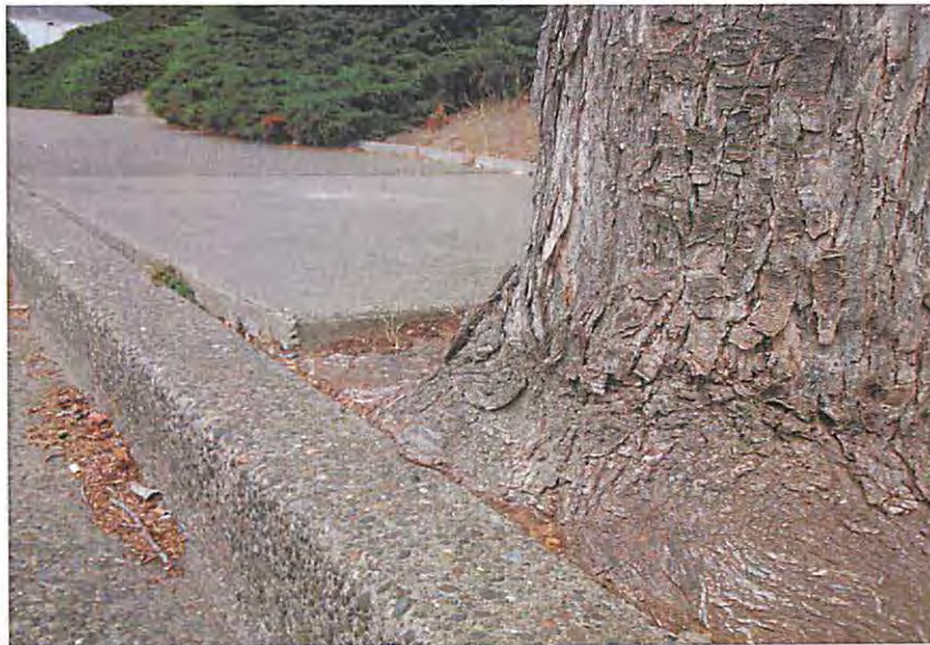
Tree root damage caused to sidewalk
