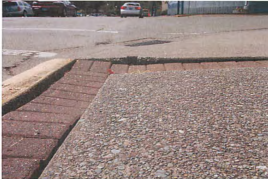
Brick separation along tree wells.
