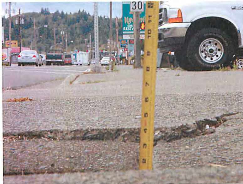
Vertical separation along cracks
