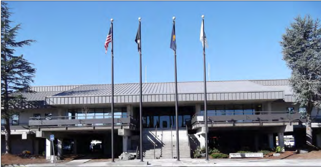
City Hall Seismic Upgrade
