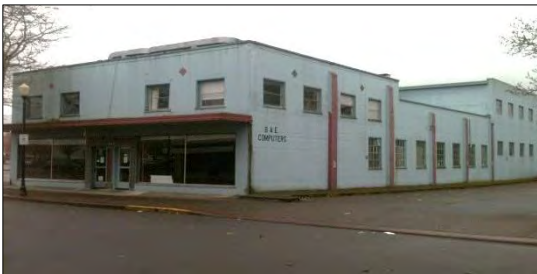
Ford Building (Before)
