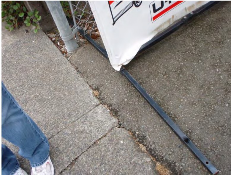
Vertical separation at the score line.
