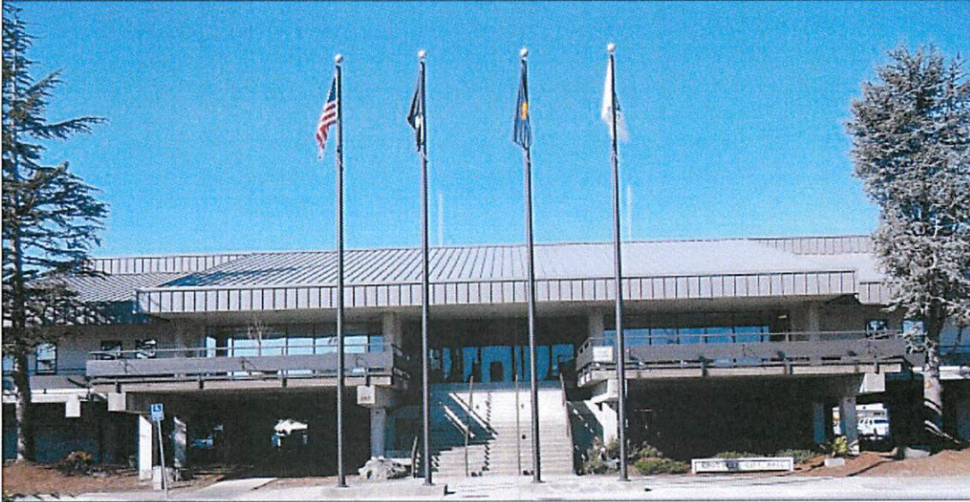
City Hall Seismic Upgrade
