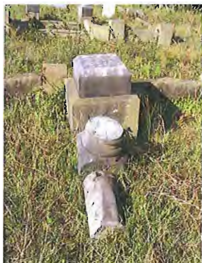
Vandalized headstone in need of repair - old mortar loosens and headstones often break along these joints.
