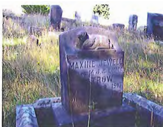
Headstone of Maxine Jewell Ostrow, showing discoloration and loss of patina from improper cleaning with a wire bristle brush.
