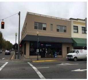
Building Name: HGE Building Address: 333 S 4<sup>th</sup> Street URA Funds: \$25,000 Value of Improvement: \$51,800 Project Completed: August 2016 Description: Cleaned, repaired and painted the exterior, replaced windows and doors, added gutter/downspouts, exterior lighting, minor restoration of stone veneer, replaced the entry door.
