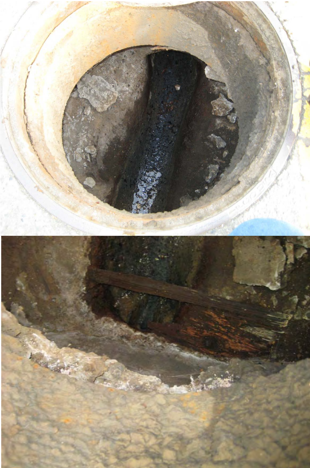
Figure 1.2.4 – Discharge Manhole and Hydrogen Sulfide Evidence
