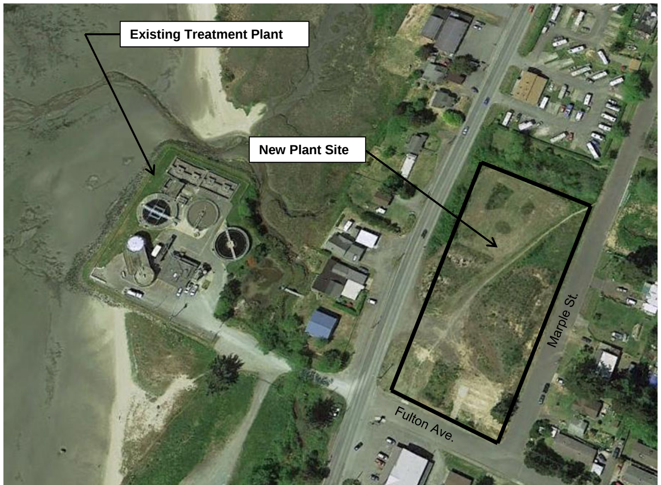
Figure A-1 – Site Location
