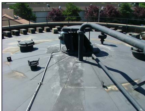
Primary Digester Floating Cover
