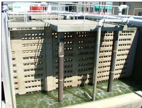
Dewatered Aeration Basin
