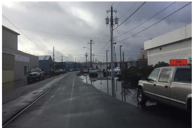
Seasonal inundation from the Bay creates localized flooding along Front Street.
