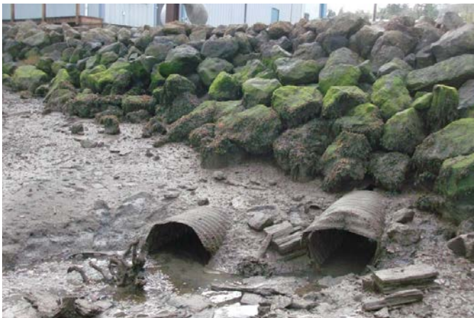
Inadequate and aging stormwater infrastructure needs upgrades. Credit: Aaron Speakman
