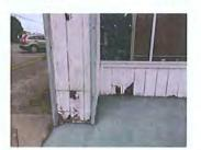
A6. The recessed area on the west elevation (Wall Street) will be framed in and sided with the same Hardie product as the south elevation. The south and west elevations will be painted a medium warm Grey.
