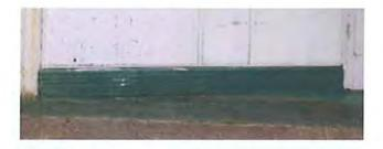
A5. The deteriorated T1-11 siding on the south elevation will be removed and a Hardie product that resembles stucco will be installed.
