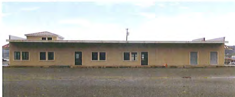
West elevation (photo taken December 29, 2014)
