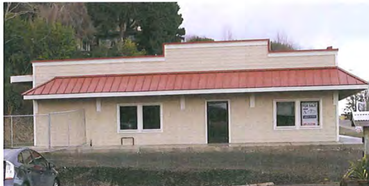
South elevation (photo taken December 29, 2014)
