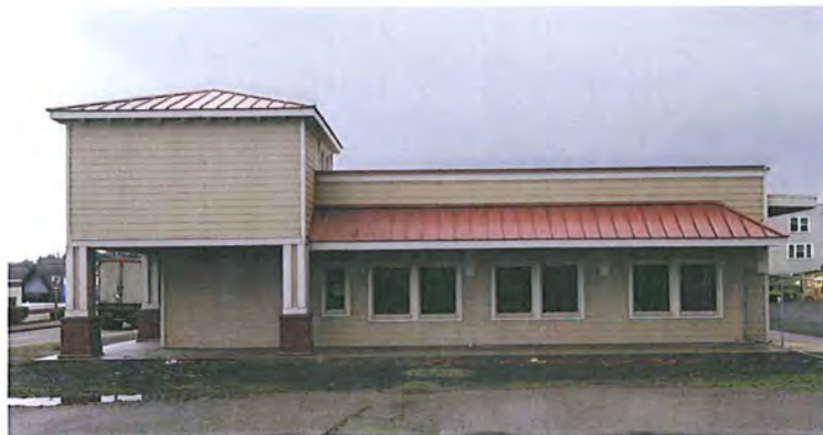
North elevation (photo taken December 29, 2014)
