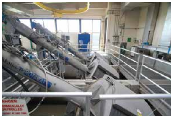
Figure 6-3: Rotating Drum Screen
