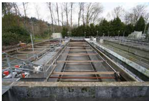
Figure 6-6: Example of Rectangular Primary Clarifier
