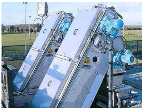
Figure 6-2: Perforated Plate Screen
