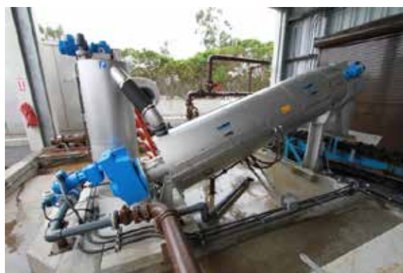
Figure 6-9: Example of Dewatering Screw Press
