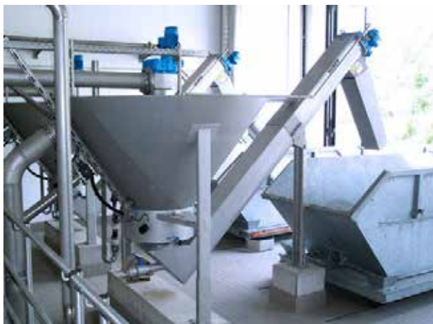
Figure 6-5: Example of Grit Washing System (Huber)
