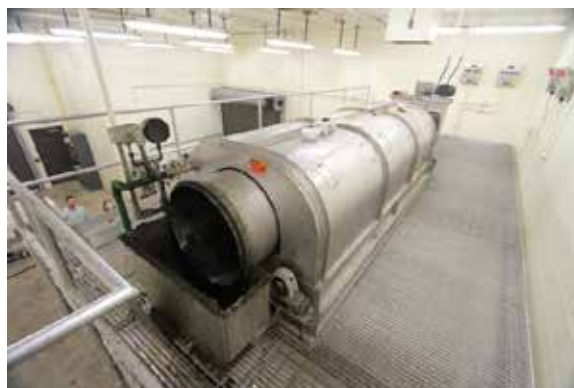
Figure 6-8: Example of Rotating Drum Thickener
