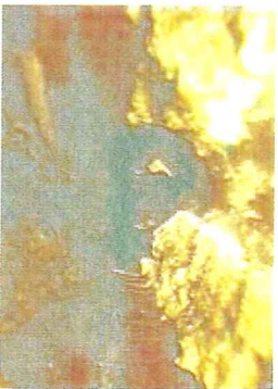
Actual photo taken by remote controlled camera showing grease buildup in sewer pipe interior.
