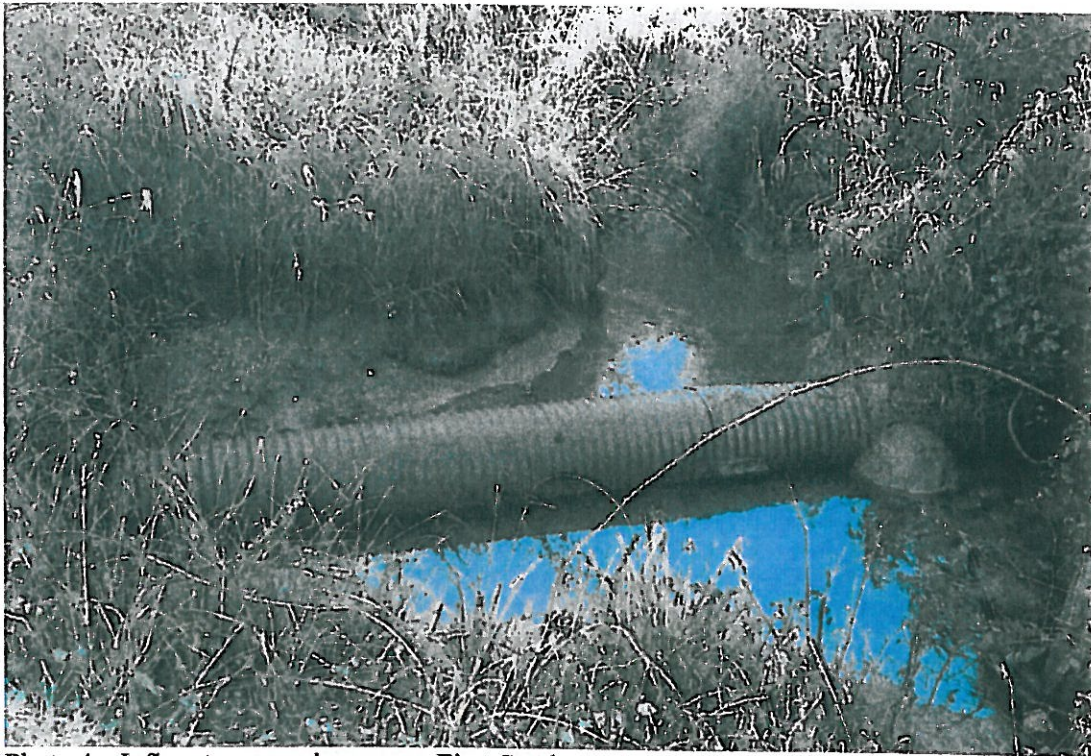
Photo 4 – Influent sewer pipe across First Creek.
