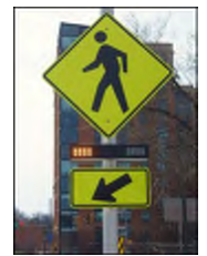
Rapid Rectangular Flashing Beacon (RRFB)
