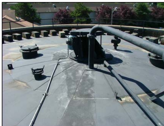
Primary Digester Floating Cover
