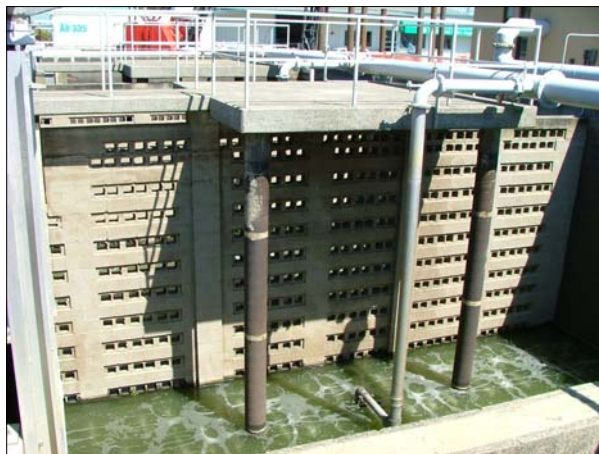
Dewatered Aeration Basin
