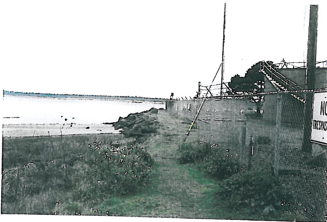
Photo 1 – Looking west at Coos Bay and the southern boundary of WWTP No. 2. Riprap protects the southern, western, northern boundaries of the site.
