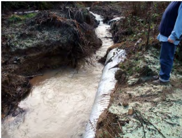
Failure of a hay bale, used as an erosion control device, that became lodged in a culvert and resulted in the stream cutting through the road.
