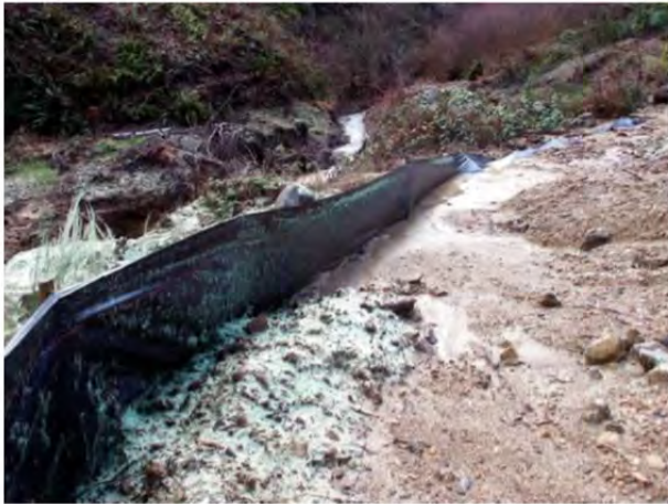
Silt fence overtopped by eroding soil during construction of the Coos County pipeline in 2003 and discharged sediment into a tributary of the Coquille River.
