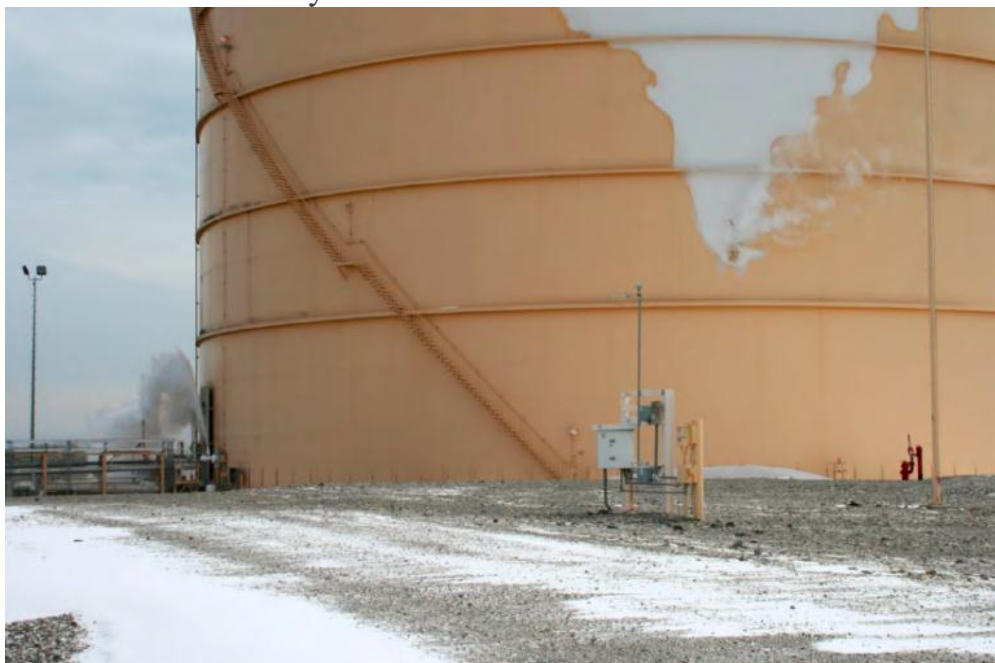
A V-shaped ice formation develops above the puncture on Plymouth LNG tank while pipe (lower left) spews LNG and gas vapor. By Washington Utilities and Transportation Commission (Used with permission.)
